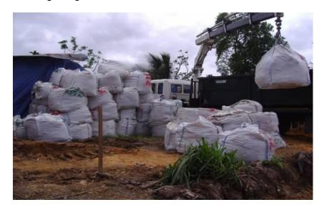
\* Based on XRF determinations the bags were labelled appropriately i.e. lead contaminated soil <1000ppm and those > 1000 ppm.
